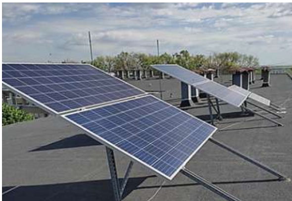
Fig. 2. Photos of four SPs mounted permanently on the roof of the laboratory in the University facing south with an angle of inclination of up to 45^{\circ}
